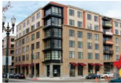
Appropriate: Change of materials and step back above four floors (Image: Crandall Arantula)
