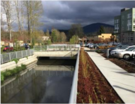
Inappropriate: Parking located between buildings and natural area (Image: Crandall Avambula)
